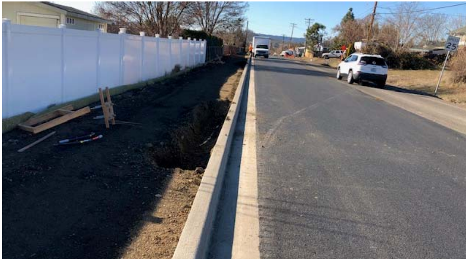
Final Paving from Bridgeport Dr. to Robert Trent Jones Blvd.
