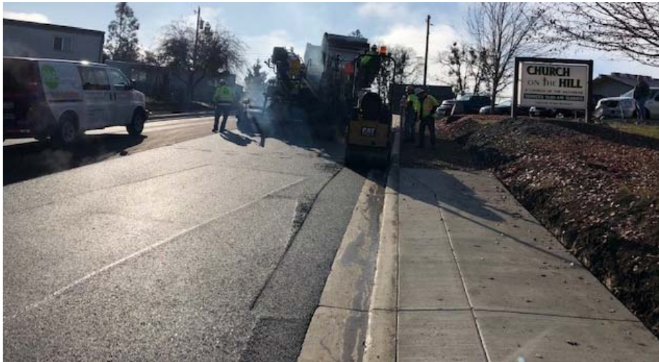
Final Paving of Stevens Road
