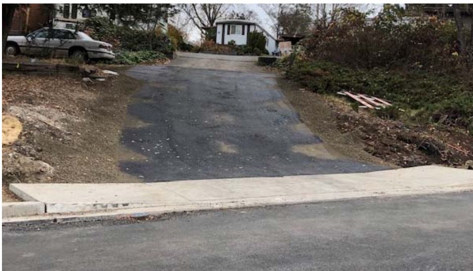
Concrete driveways were completed.
