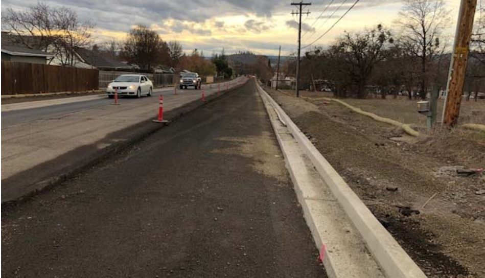
Widening was completed for Stage 2.
