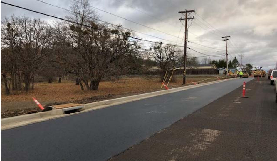
Base lift paving.
