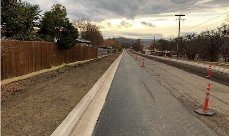
Base lift paving.
