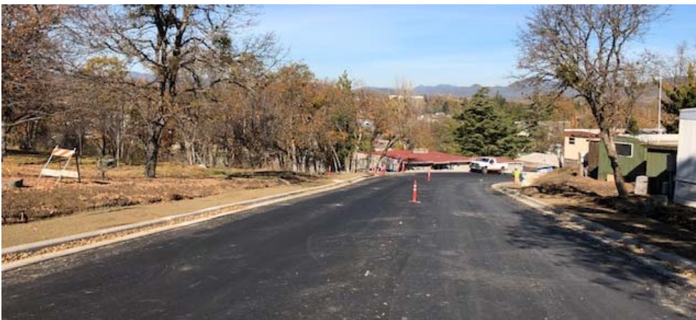
Temporary striping is scheduled for Monday, November 4, 2019.
