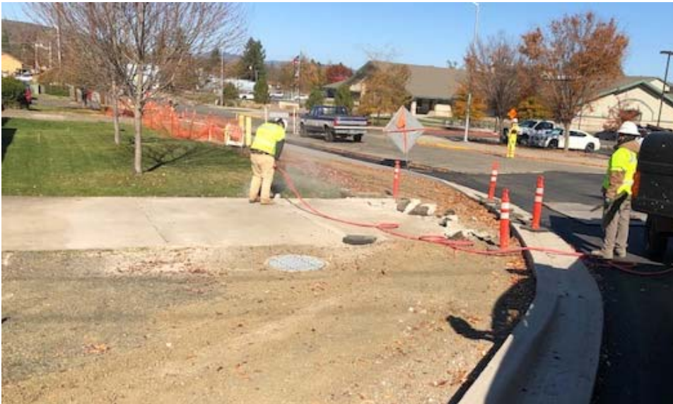
Driveway preparation is underway.
