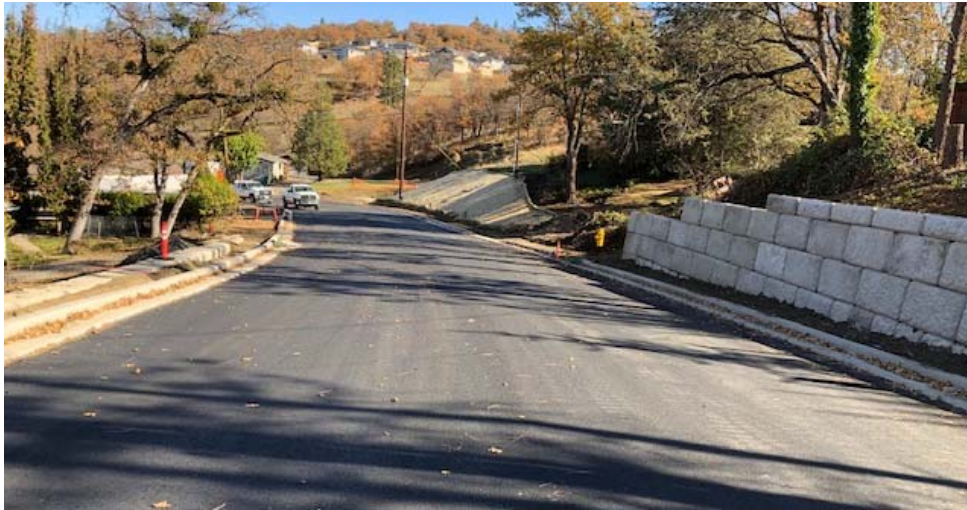
Base paving was completed for Stage 1.
