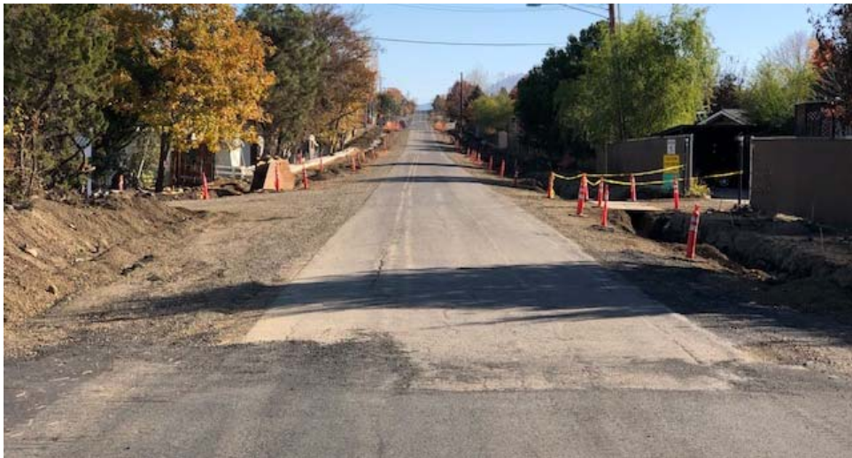
Widening for Stage 2 continues (Idlewood Drive to Robert Trent Jones Boulevard).
