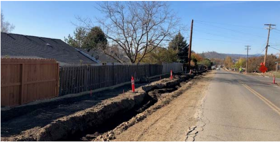
Conduit installation for new lighting.
