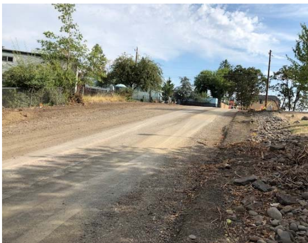
Stage 1 pavement removed.
