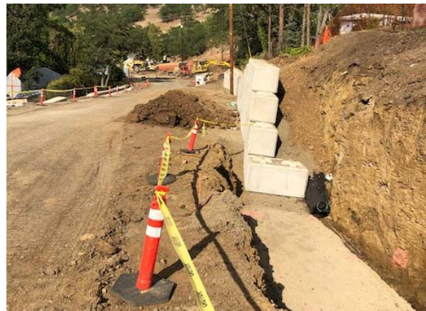
The Ultrablocks were delivered to the site, and unloaded directly by Knife River Materials on Main Street. This saved time and effort for both the City and Knife River.
