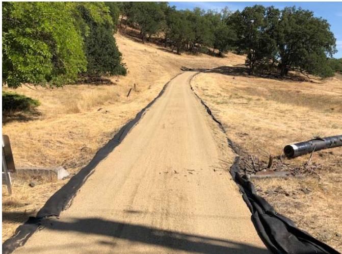
Onyx Road temporary pedestrian detour.
