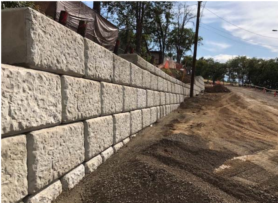
Retaining Wall "B" Construction.
