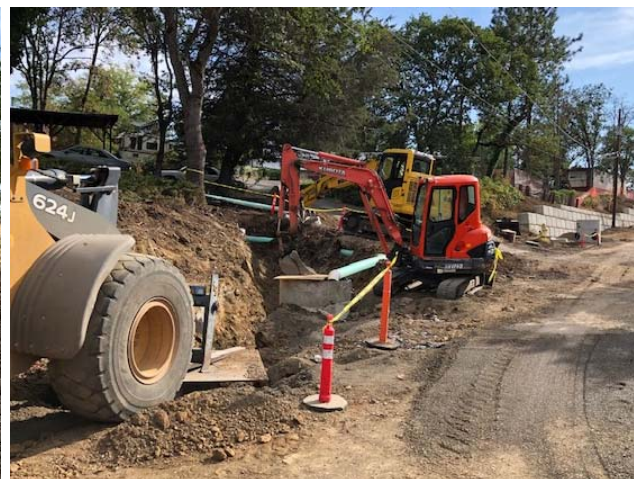
Relocation of the RVSS manhole continues.
