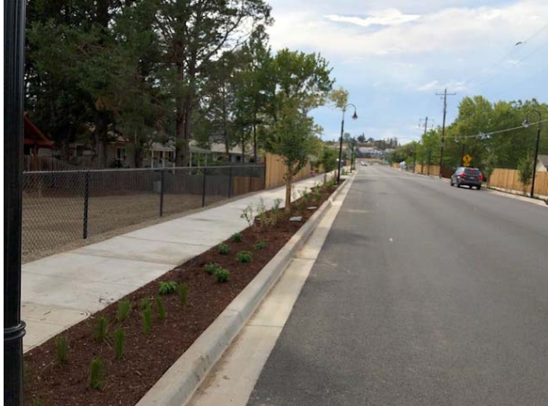
Completed fences and planters.
