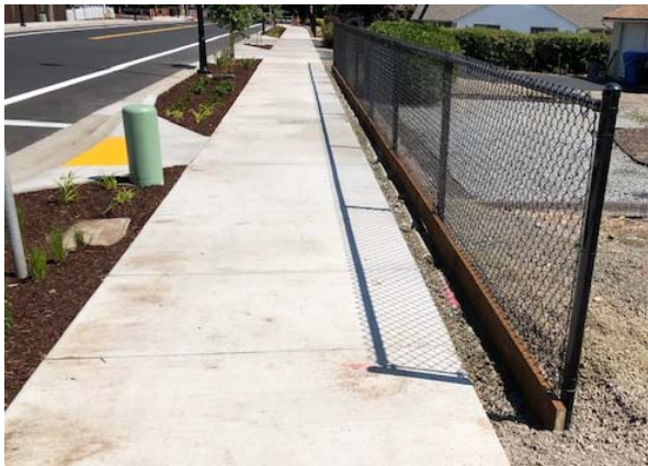
Rock backing was placed adjacent to fences.
