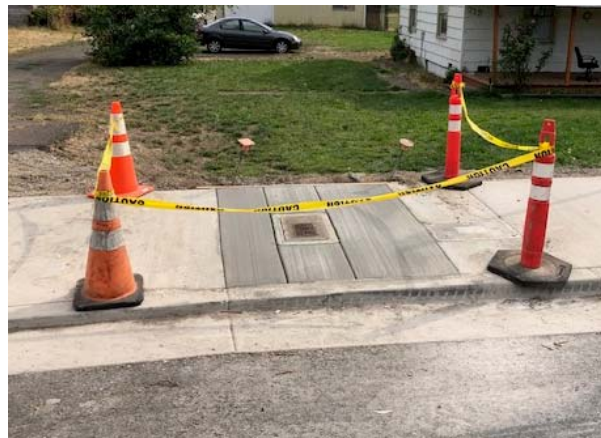
Cracked concrete panels were replaced.
