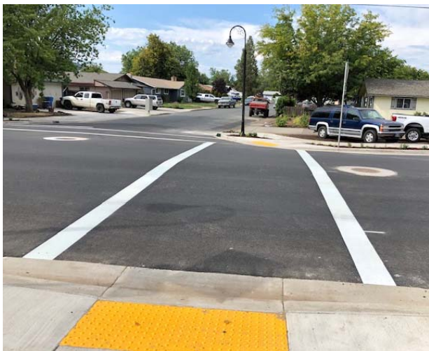
Crosswalks were completed.
