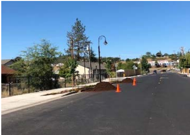
Mulch was placed in the planters.
