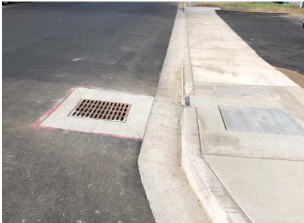
Drainage tie ins were completed.
