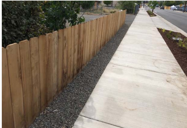
Cracked concrete panels were replaced.
