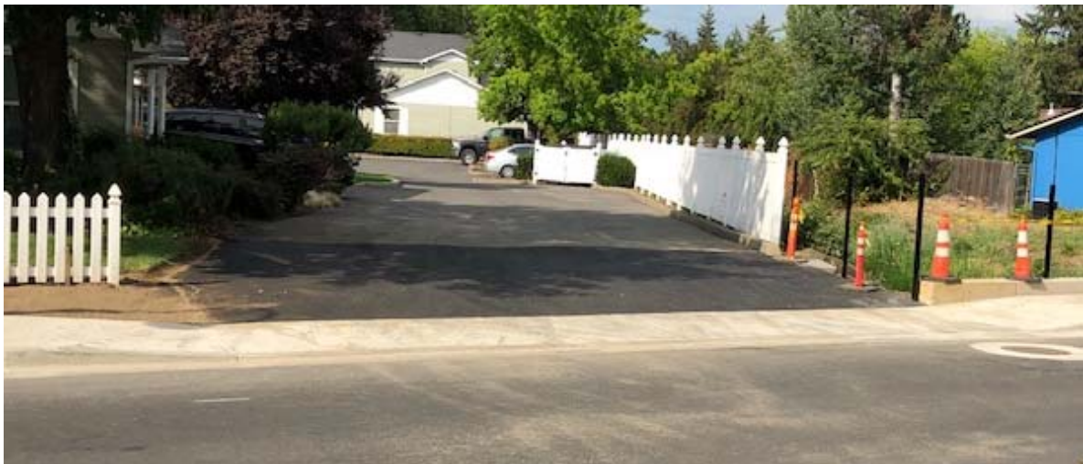
The last driveway was paved.
