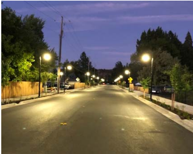
Lighting was installed.
