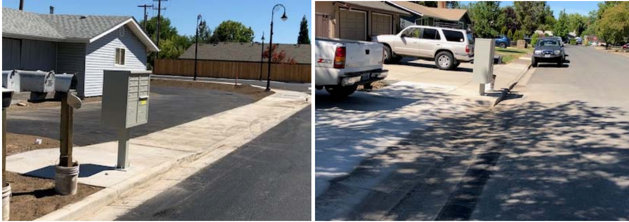
Cluster mailbox units were installed.
