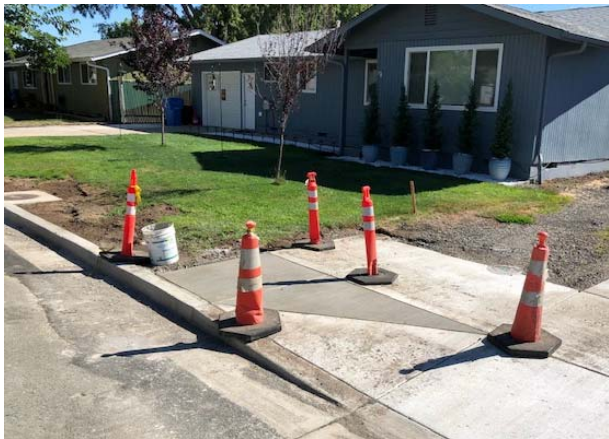
Concrete panel for mailboxes.
