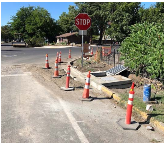
The last water quality structure was installed.
