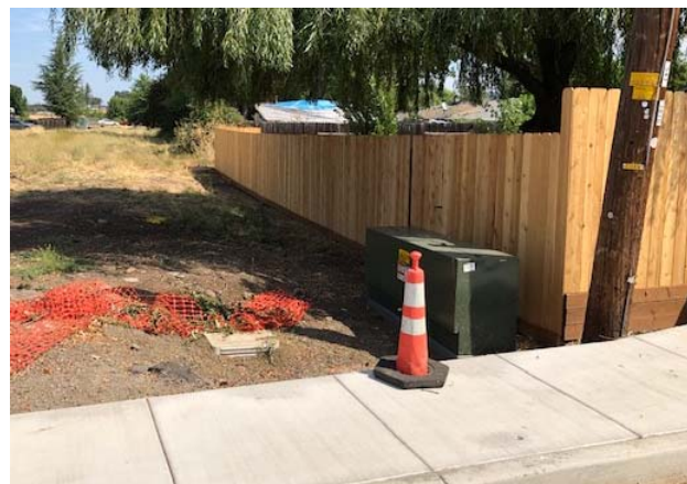
Fencing was installed by Quality Fence.
