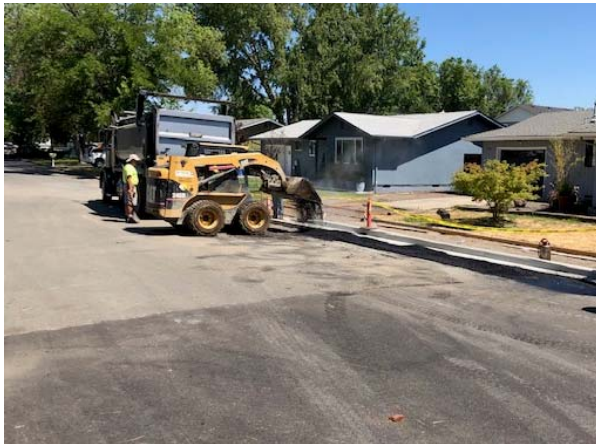
Drainage tie ins were completed.
