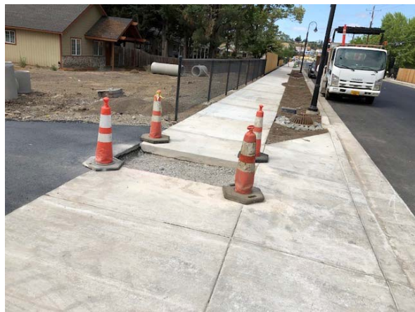
Cracked concrete panels were replaced.
