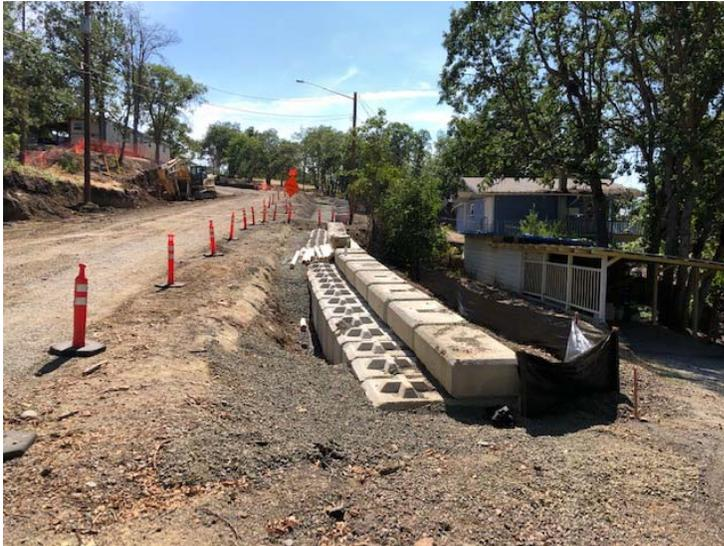
Installation of the Ultrablocks for Wall "A" was completed.
