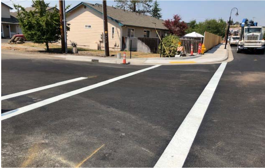
Work began to place the vinyl crosswalk striping.
