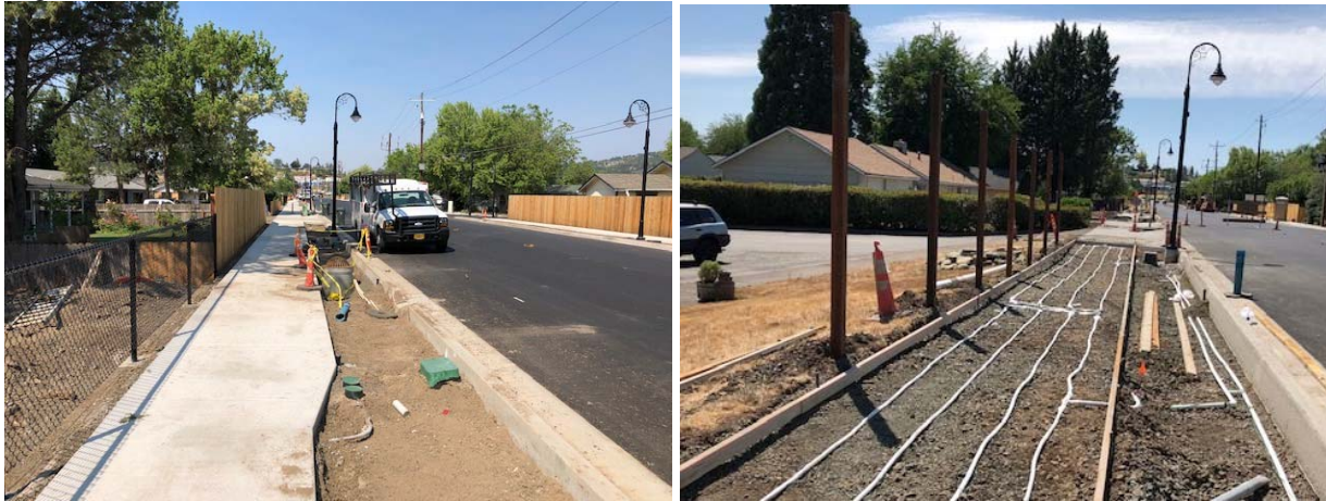
Overstreet Hydroseeding completed the last irrigation connections.
