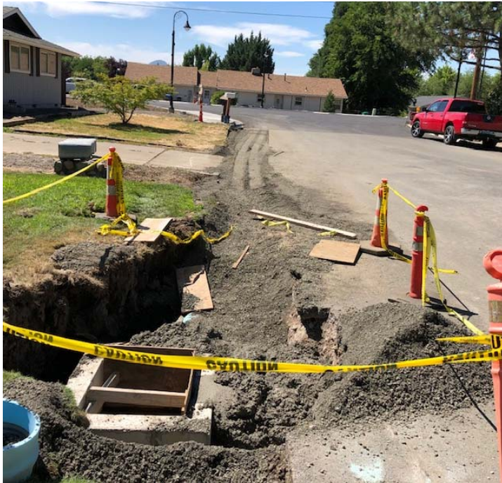
Drainage ties ins were completed on the side streets.
