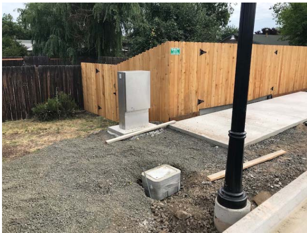
Irrigation controller box installed.
