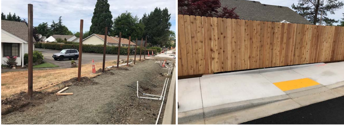
Quality Fence installed additional fences/supports for the project.
