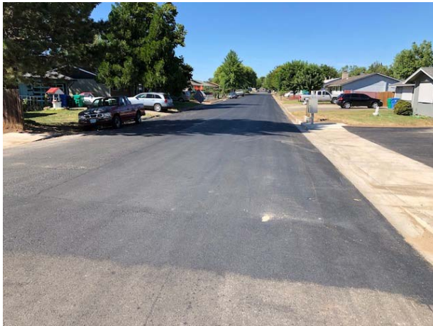
Completed Seal Coat.
