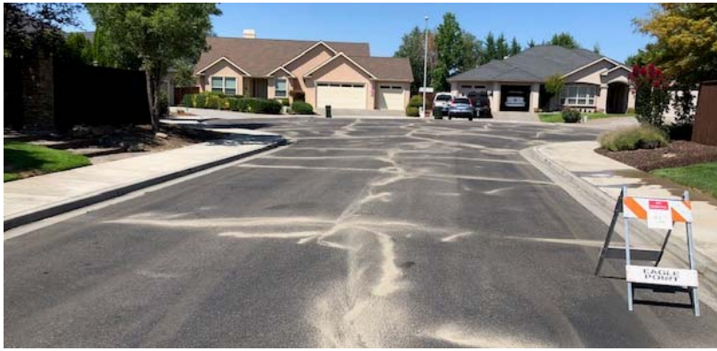
Completed Crack Seal project.
