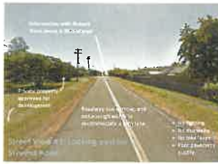
Stevens Road Improvement Project Eagle Point, OR
